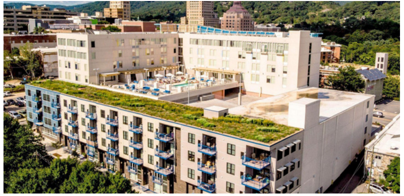
Photo: Garage Apartments 2019. Photo: Living Roofs, Inc.
