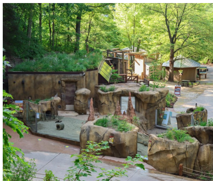
LAPT Platinum Certified green roof at the John Ball Zoo in Michigan
