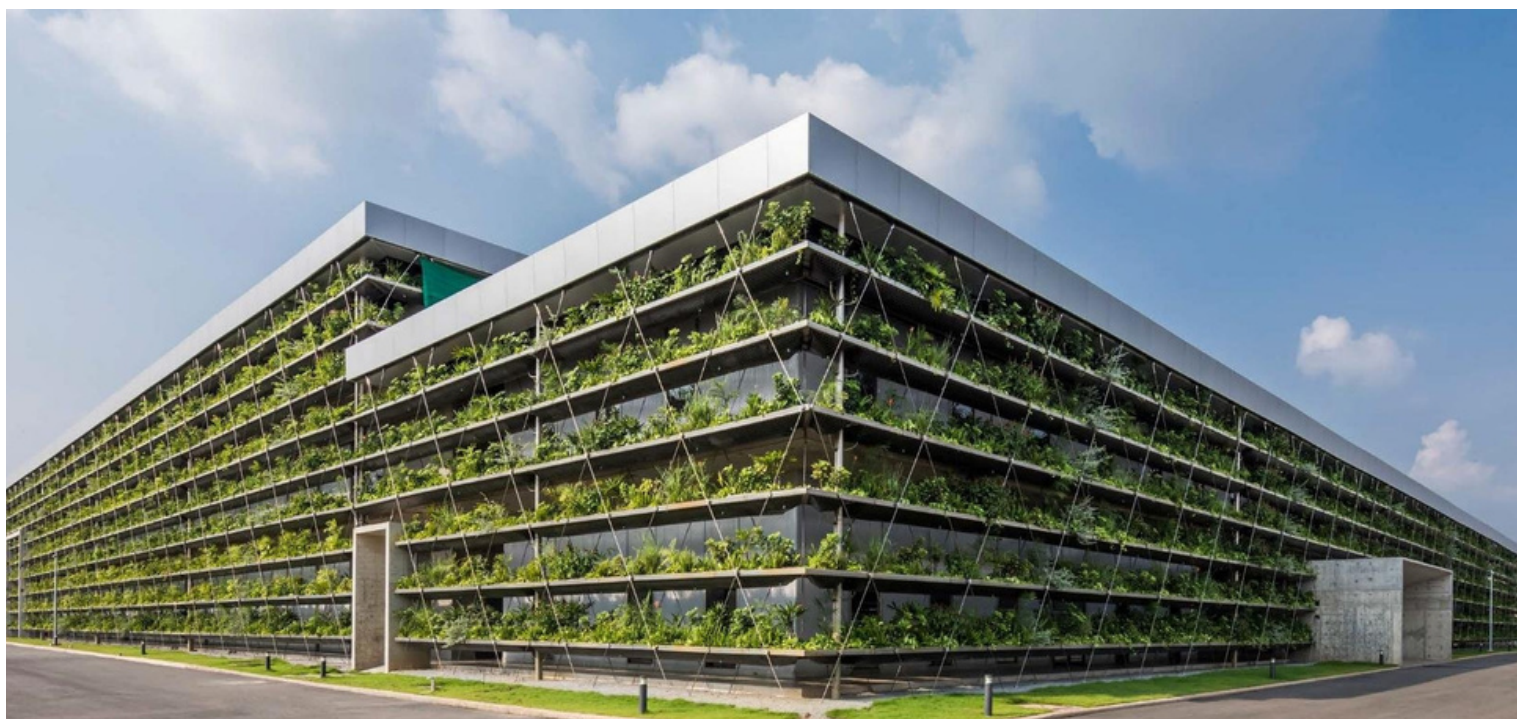
Multi-story green facades around an inner courtyard, Jakob Rope Systems, Vietnam. Photo: Oki Hiroyuki for G8A Architects, HCMC, Vietnam
